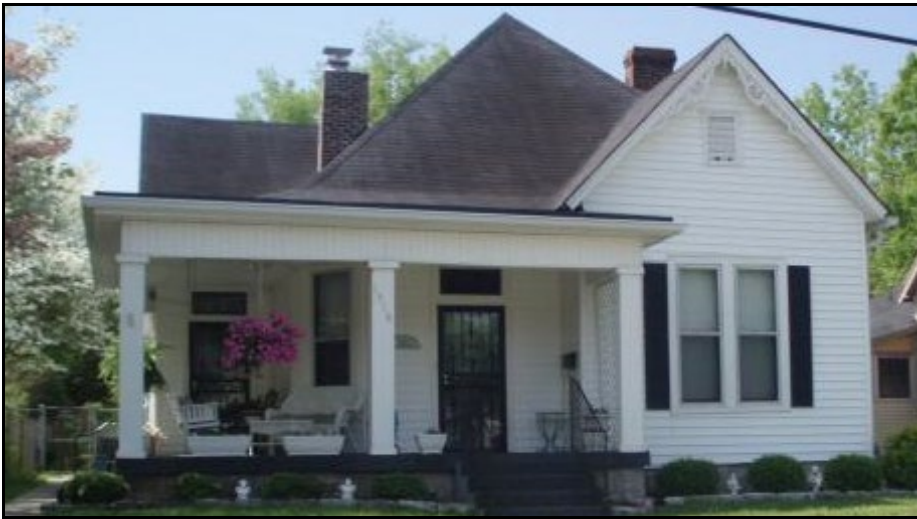
1516 Fatherland Street. Staff measured as ~22ft from grade to front gable
