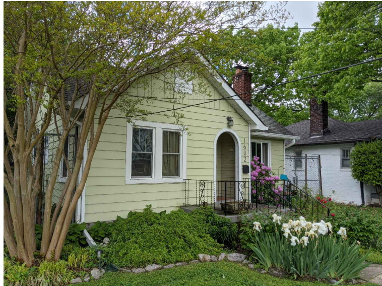
EXISTING CONDITIONS PHOTOS
