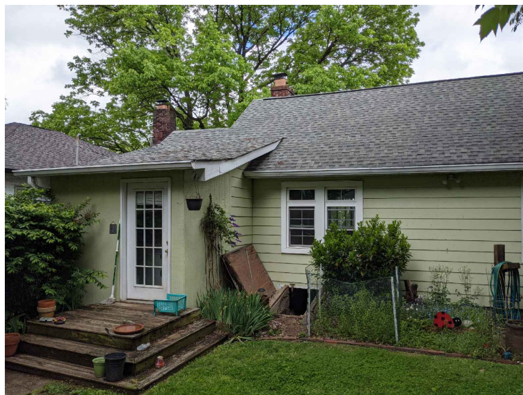
EXISTING CONDITIONS PHOTOS
