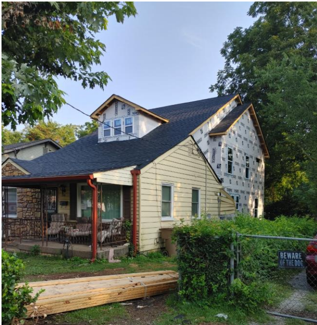
Figure 1: Front-right, as constructed.
