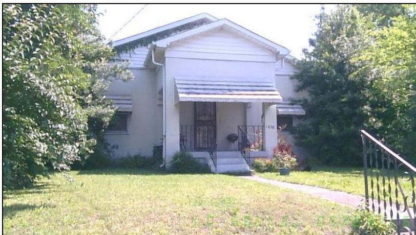
Figure 1. 1826 5 th Avenue N.
