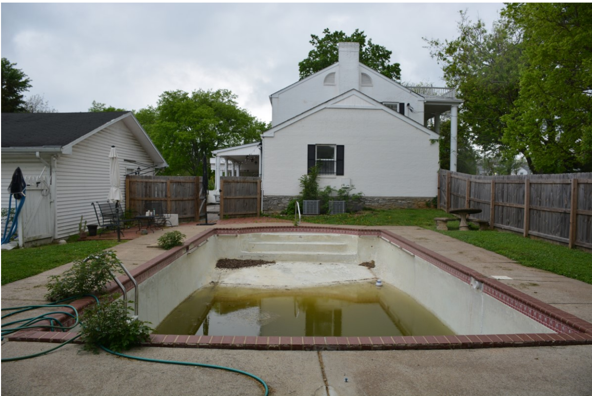
Pool looking towards left side of house.
