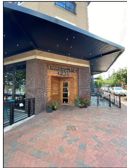
Figure 2: Sign above entrance.
