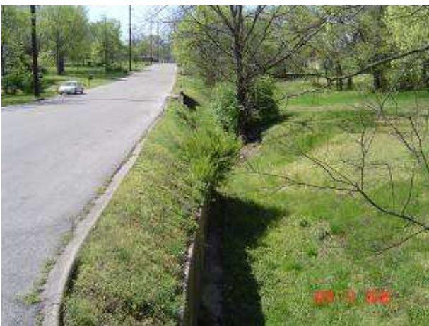
Fig. 2. Southerly view of western margin of McGavock Pike (Photo taken by J. Honeycutt, MPW)
