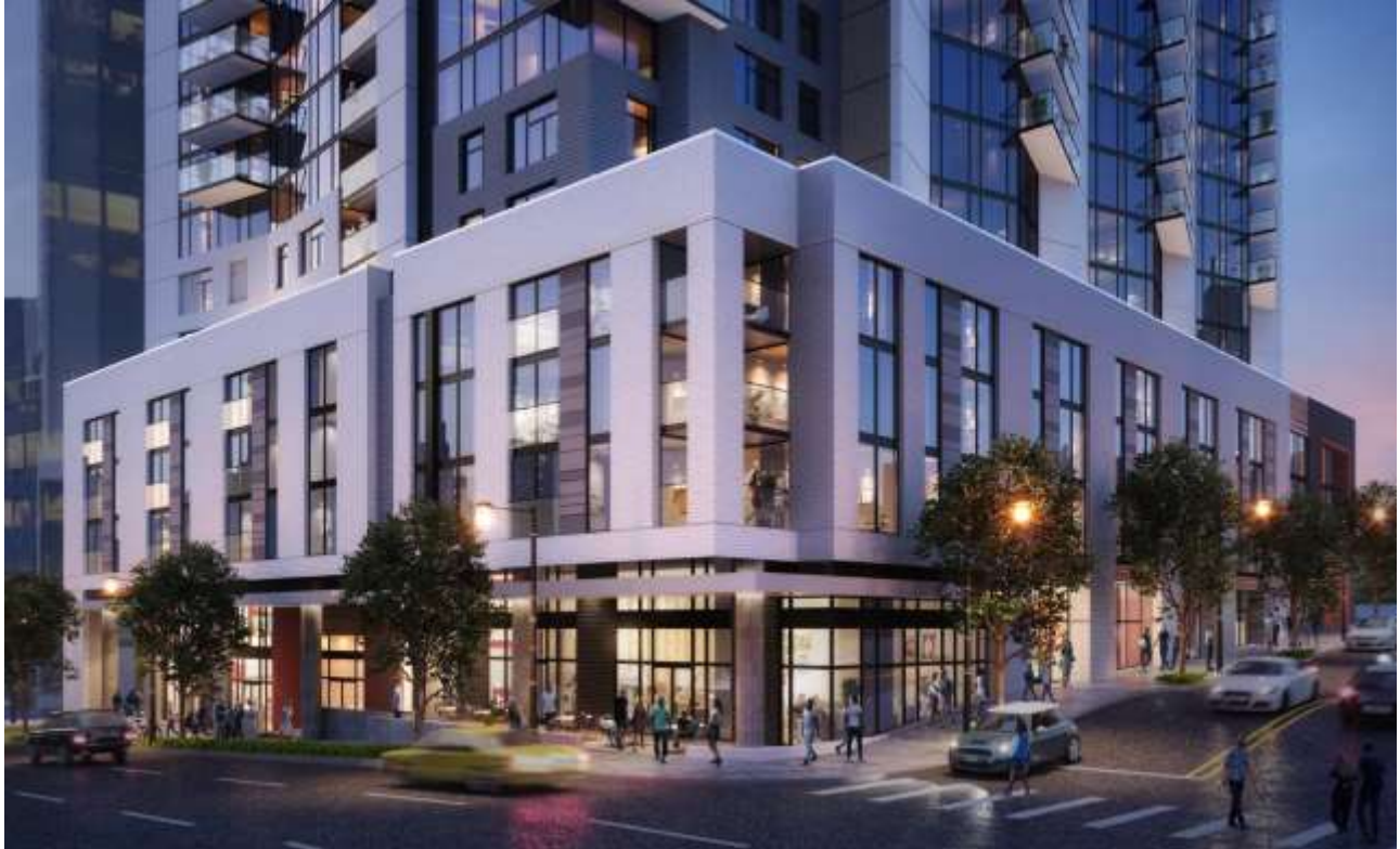
Figure 5: View from intersection of 13th Avenue South and McGavock Street showing an active streetscape from the covered arcade and retail activation
