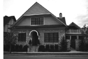
Front Elevation All Buildings To Be Primarily Brick and Stone and Other Masonry Products (No Vinyl). Buildings are Encouraged To Have Front Porch Entrances That Are Elevated Above the Street
