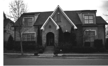
Front Elevation All Buildings To Be Primarily Brick and Stone and Other Masonry Products (No Vinyl). Buildings are Encouraged To Have Front Porch Entrances That Are Elevated Above the Street
