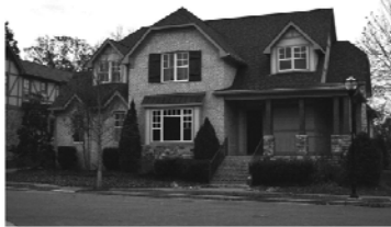
Front Elevation All Buildings To Be Primarily Brick and Stone and Other Masonry Products (No Vinyl). Buildings are Encouraged To Have Front Porch Entrances That Are Elevated Above the Street
