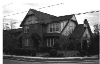
Corner Lot On Main Street All Corner Lots Shall Be Constructed To Address Each Street With A Primary and Secondary Doorway Thus Creating A Frontage Facade On Each Street. Buildings Along Church Street and Cloverland Will Set Back 20 Feet From the Right Of Way
