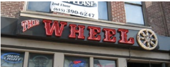
Example of raceway incorporated as sign background
