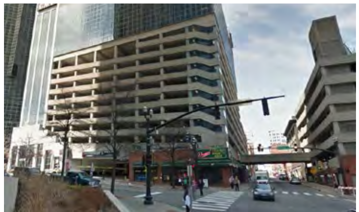
Inappropriate upper level facade treatment
