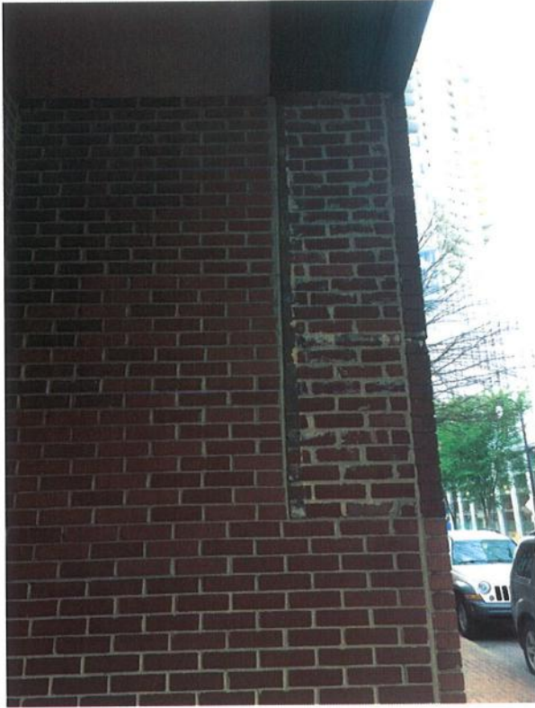
Blending of bricks from different eras due to heavy modification
