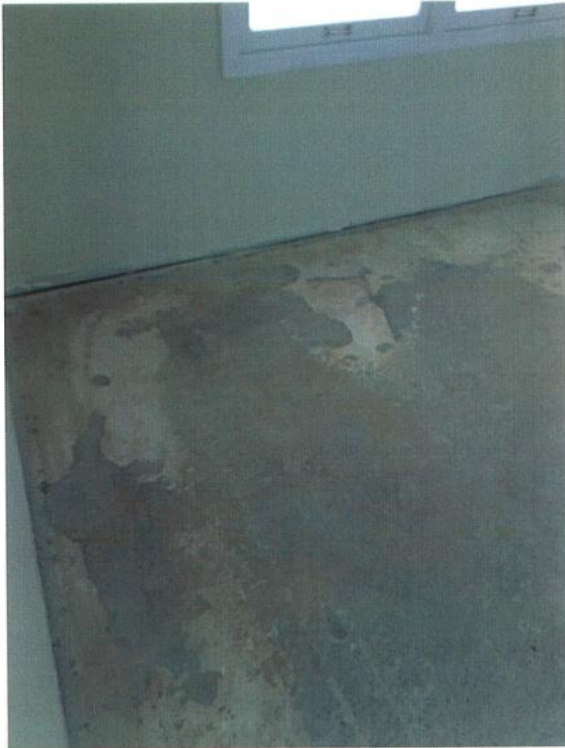
Unfinished apartment flooring
