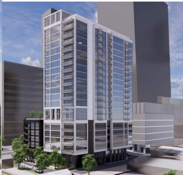
Figure 2: View of Drexel & Alley Façades
