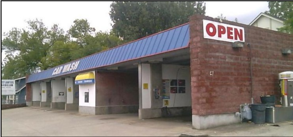
Figure 1: Existing structure at 1101 McKennie Avenue
