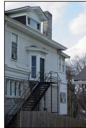
Figure 4. Existing exterior stair.
