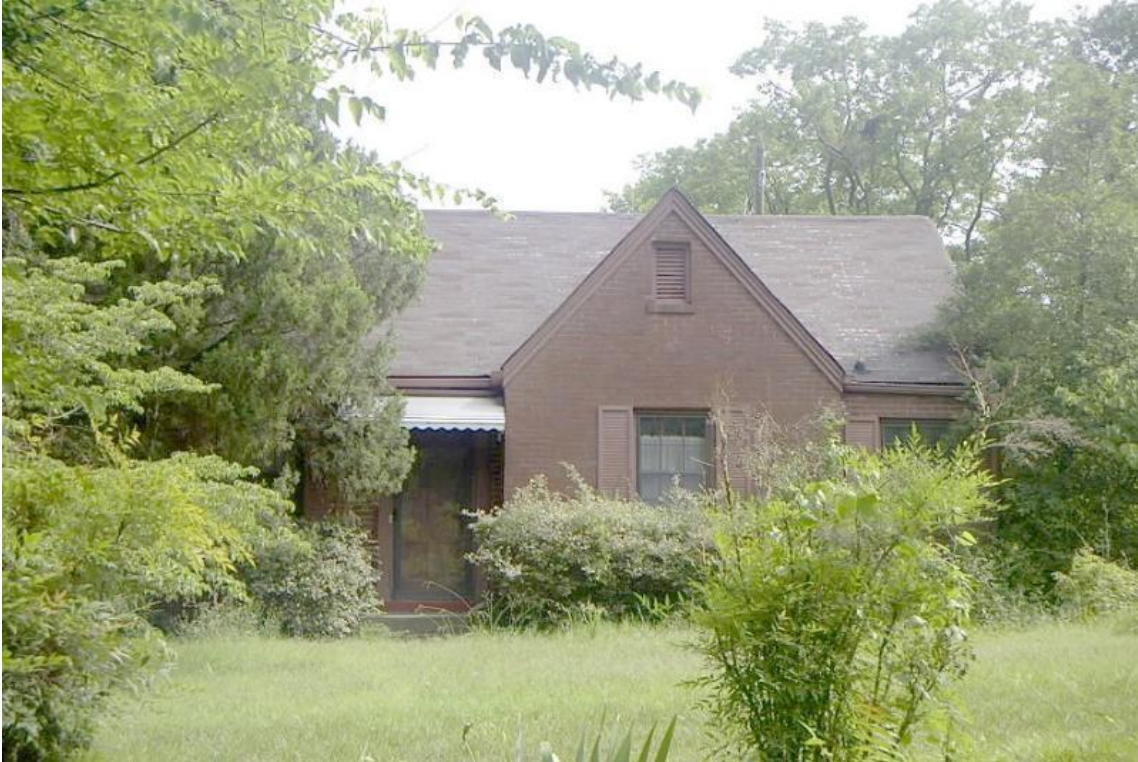
Figure 1. 2416 West Linden Avenue
