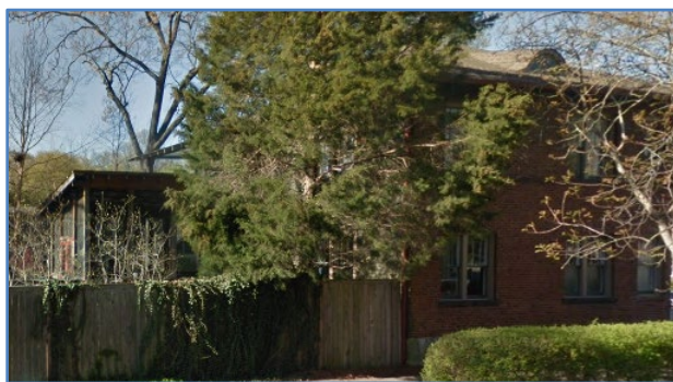
Figure 2: Existing rear screened porch to be removed.
