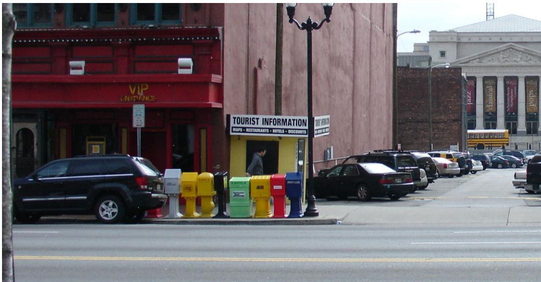
Figure 2: The subject structure in 2007.
