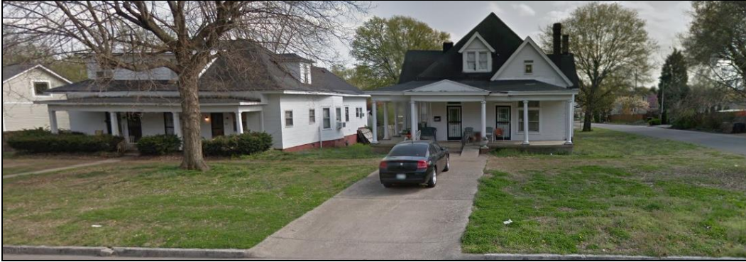
4709 and 4711 Elkins Avenue – both contributing. 4709 Elkins Ave approved for demo due to economic hardship in October 2019.
