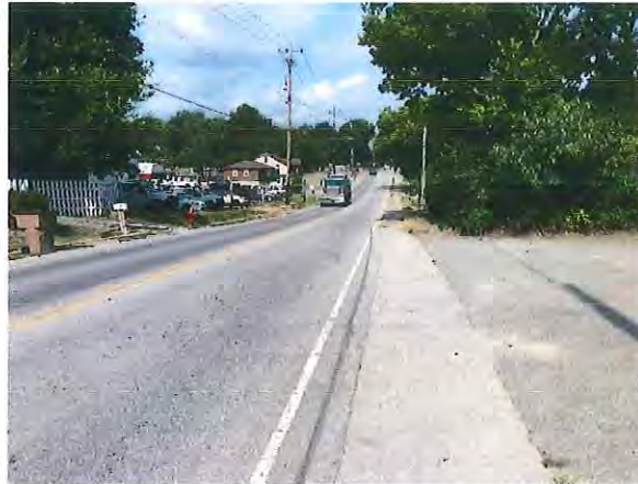
Robertson Avenue looking west, east of the project site
