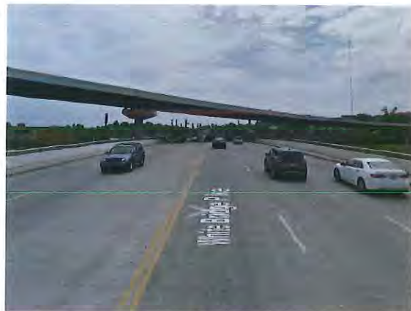
White Bridge Pike looking south, east of the project site
