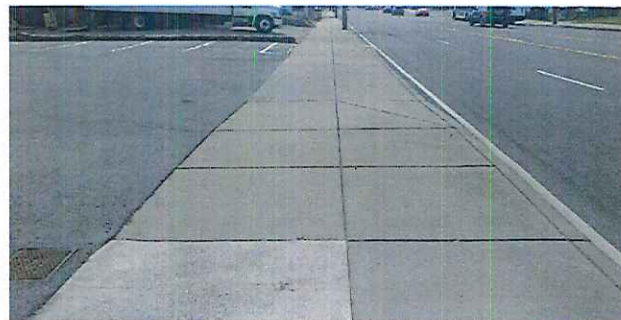
Existing Sidewalk Condition
