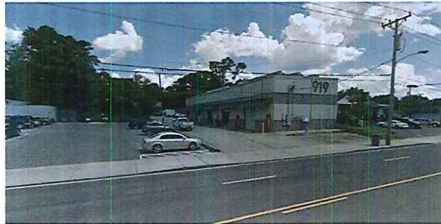
Sidewalk Connection to South Neighboring Property
