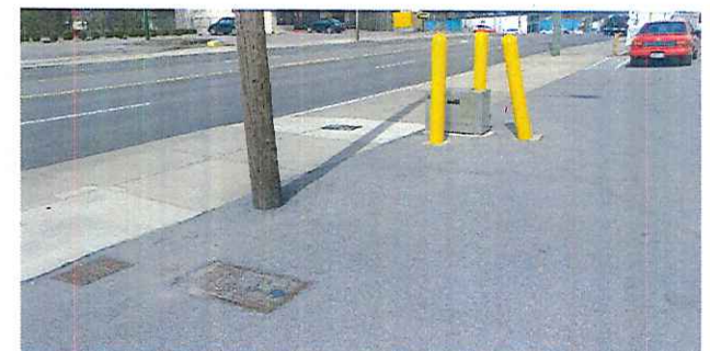
Existing Sidewalk Condition and Existing Utilities
