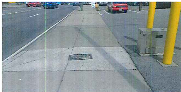
Existing Sidewalk Condition
