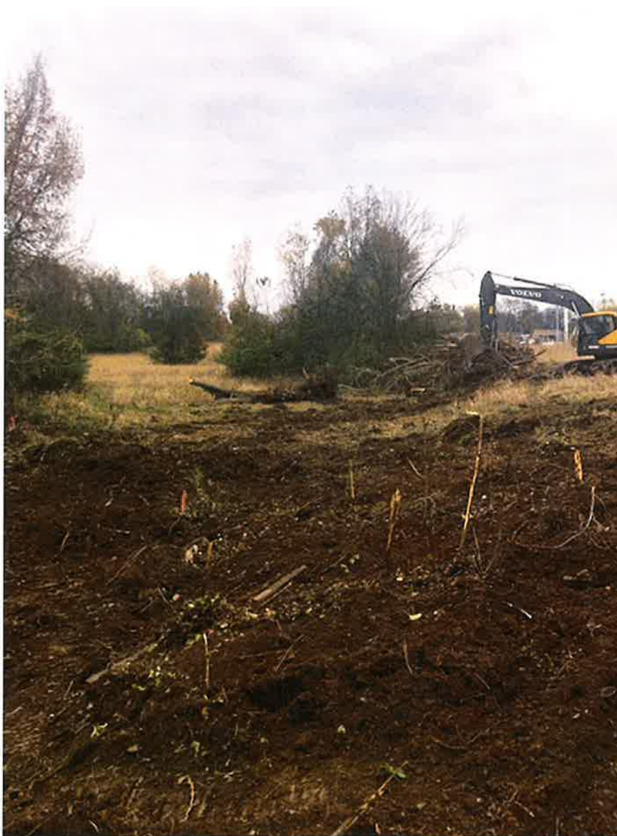
Figure 6: Conclusion of Clearing and Grading on November 11 th , 2019; view east
