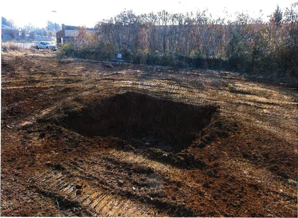
Figure 8: Excavated Compound on November 18 th , 2019
