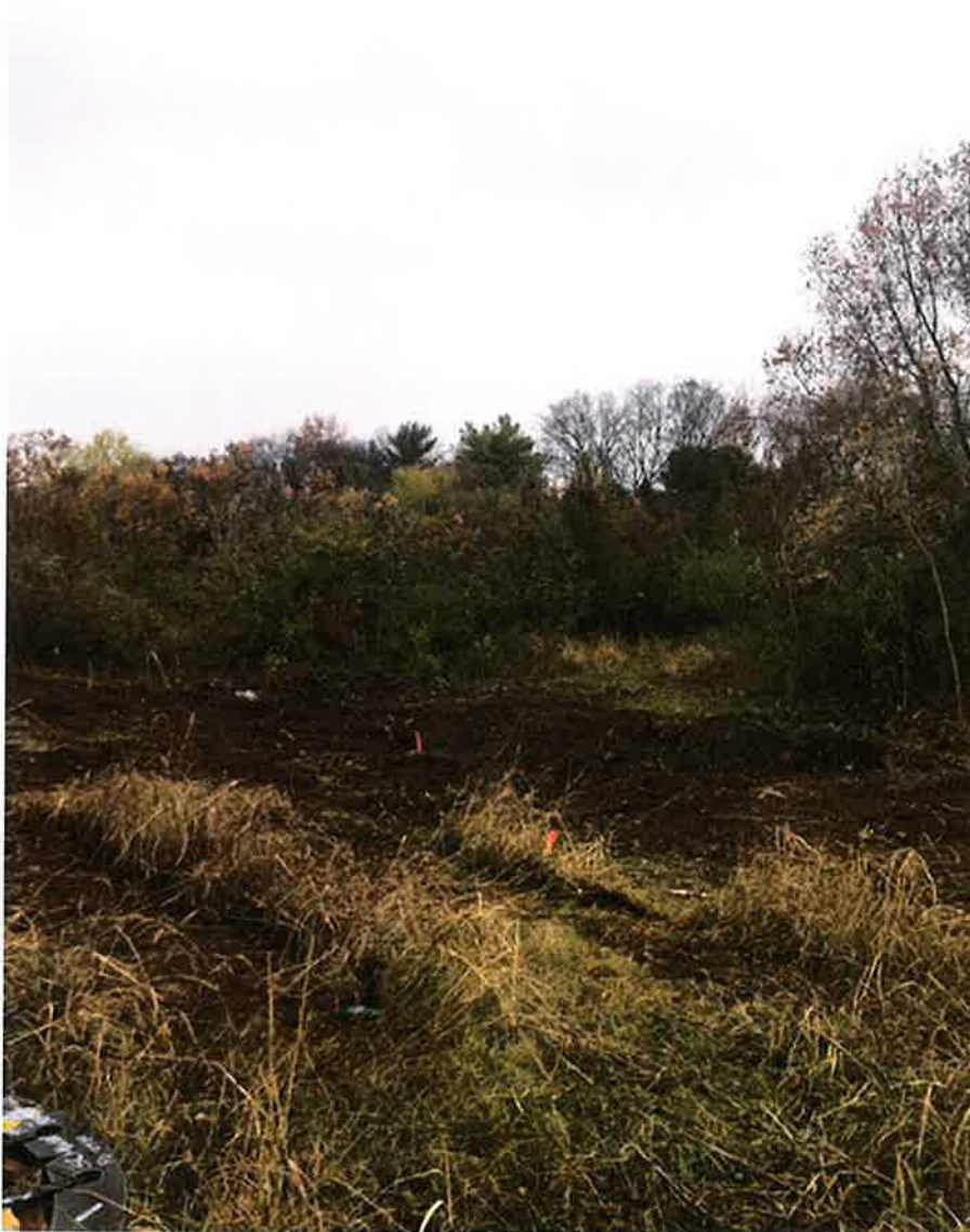
Figure 5: Conclusion of Clearing and Grading on November 11 th , 2019; view west
