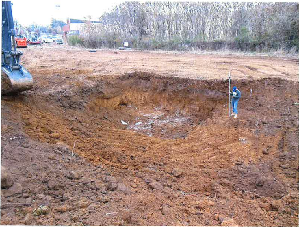
Figure 10: Extended excavation to remove extensive rock
