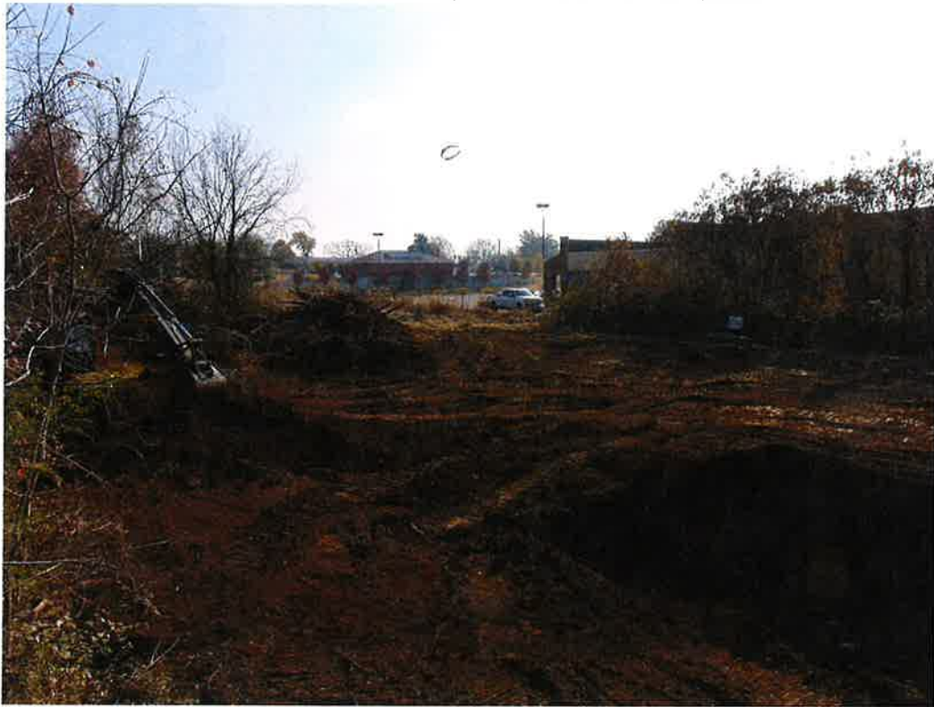
Figure 9: Cleared and graded project area on November 18 th , 2019
