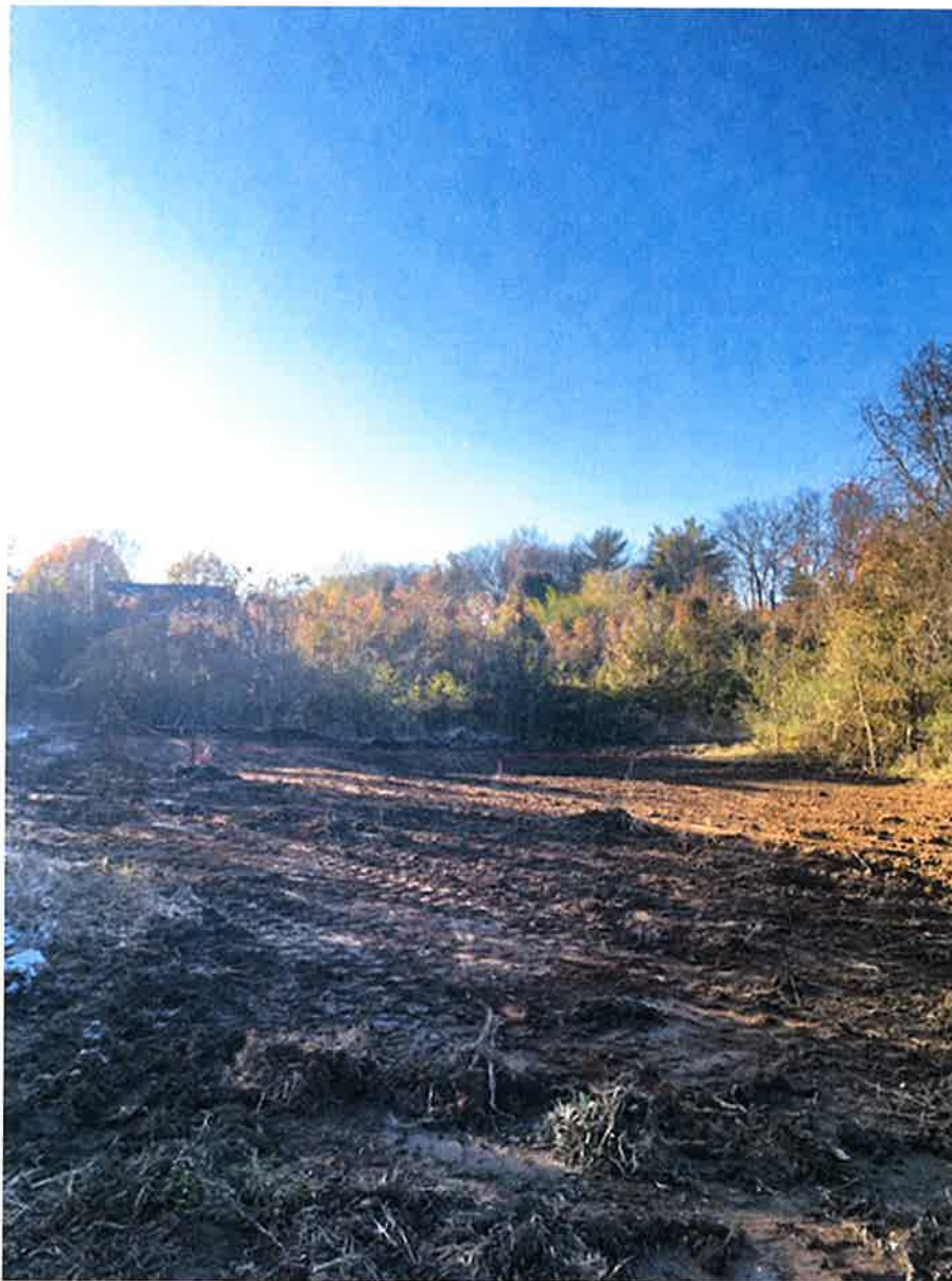
Figure 7: Conclusion of Clearing and Grading on November 12 th , 2019; view west
