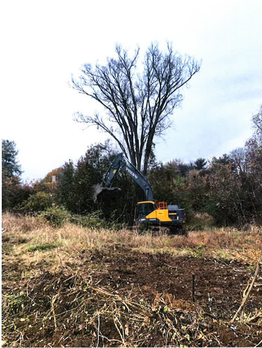
Figure 4: Excavator Clearing Major Vegetation on November 11 th , 2019; view west
