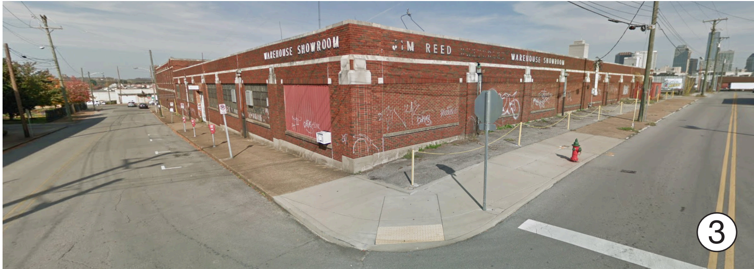
16TH AVE N at HAYES ST - Historic Coke Building
