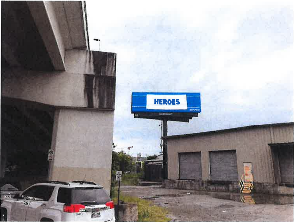
Billboard from S 1 st Street
