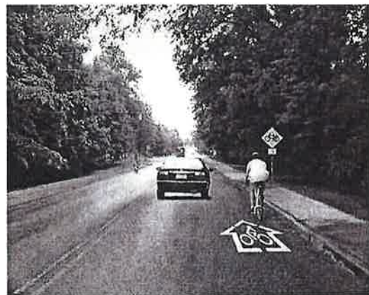
Shared roadways accommodate both vehicles and bicycles.
