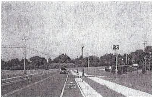
Bicycle lanes should be designed for one-way travel in the same direction as the adjacent motor vehicle traffic.
