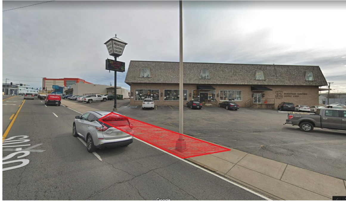
VIEW OF AFFECTED SIDEWALK ALONG LAFAYETTE STREET LOOKING SOUTH
