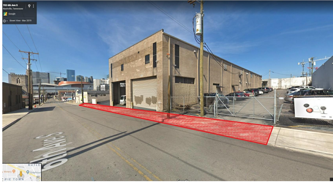
VIEW OF AFFECTED SIDEWALK ALONG 6TH AVE SOUTH LOOKING NORTH
