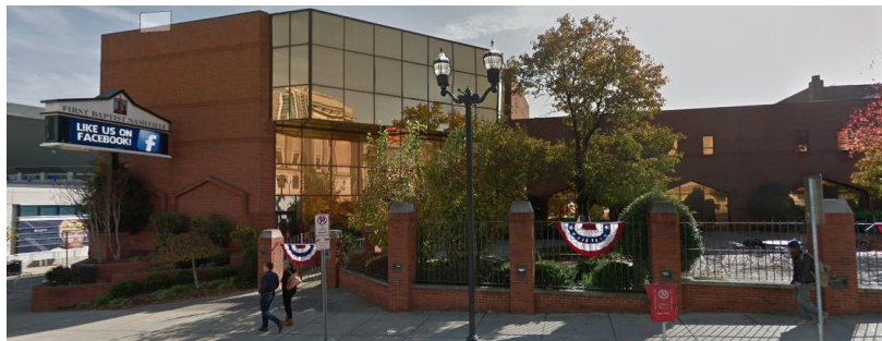
Existing Building (To Be Demolished)
