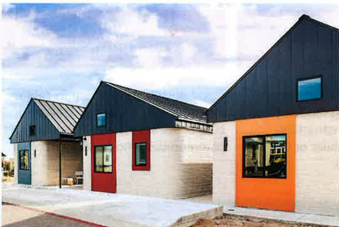
3D-printed homes in Austin, TX ICON, Logan Architecture
