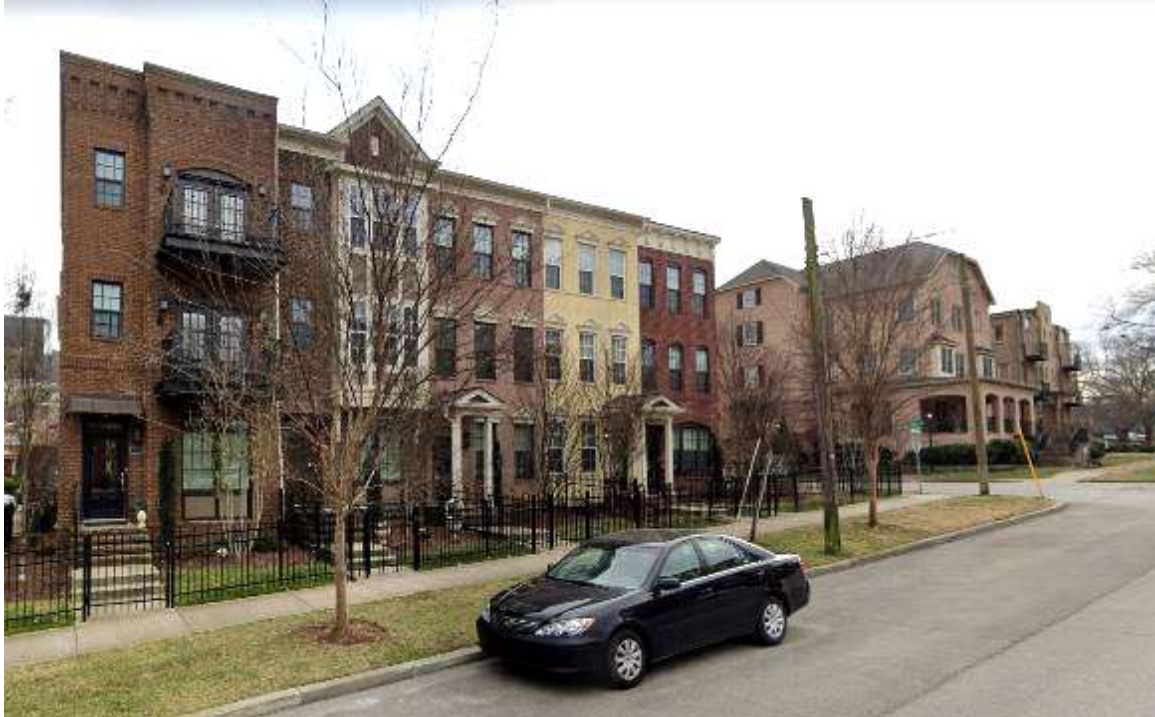
Figure 3: The townhouse development at 3145 Long Boulevard, utilizes the same staggered façade approach to deal with the irregular shaped parcel formed by Long Boulevard to the front and Belwood Street at the rear, without compromising the intent of the UDO’s setback standard.
