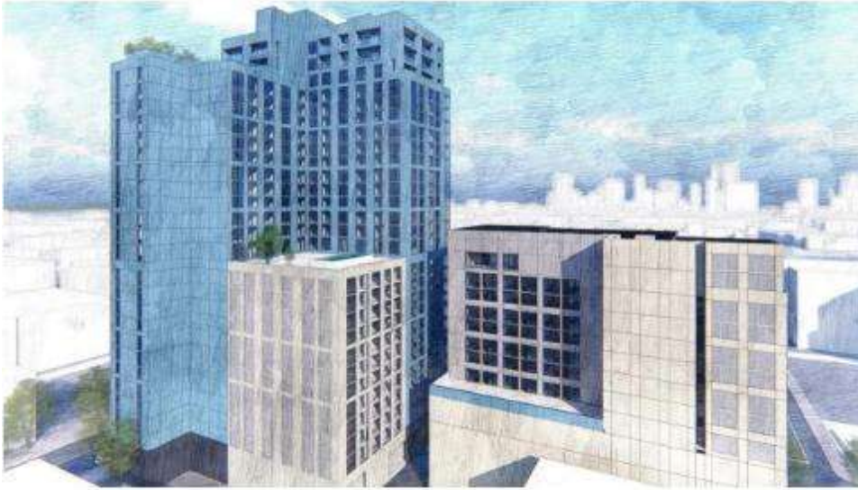
Current West-Facing Facades
