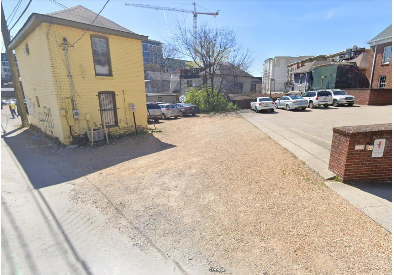
Figure 8. Unimproved Alley #456 is 9 ft wide and about 71 ft long in this gravel area.
