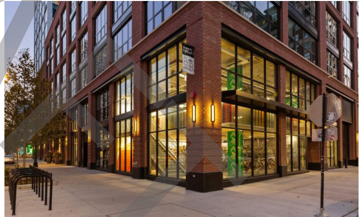
07E: "Inverted U" bicycle racks are located on the sidewalk for short-term bicycle parking, while an interior bicycle storage room allows for more secure, long-term parking.
