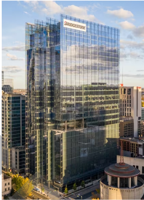
04D: Parking levels, at the Bridgestone Tower (SoBro) are screened from view with materials that fit seamlessly into the tower design.
