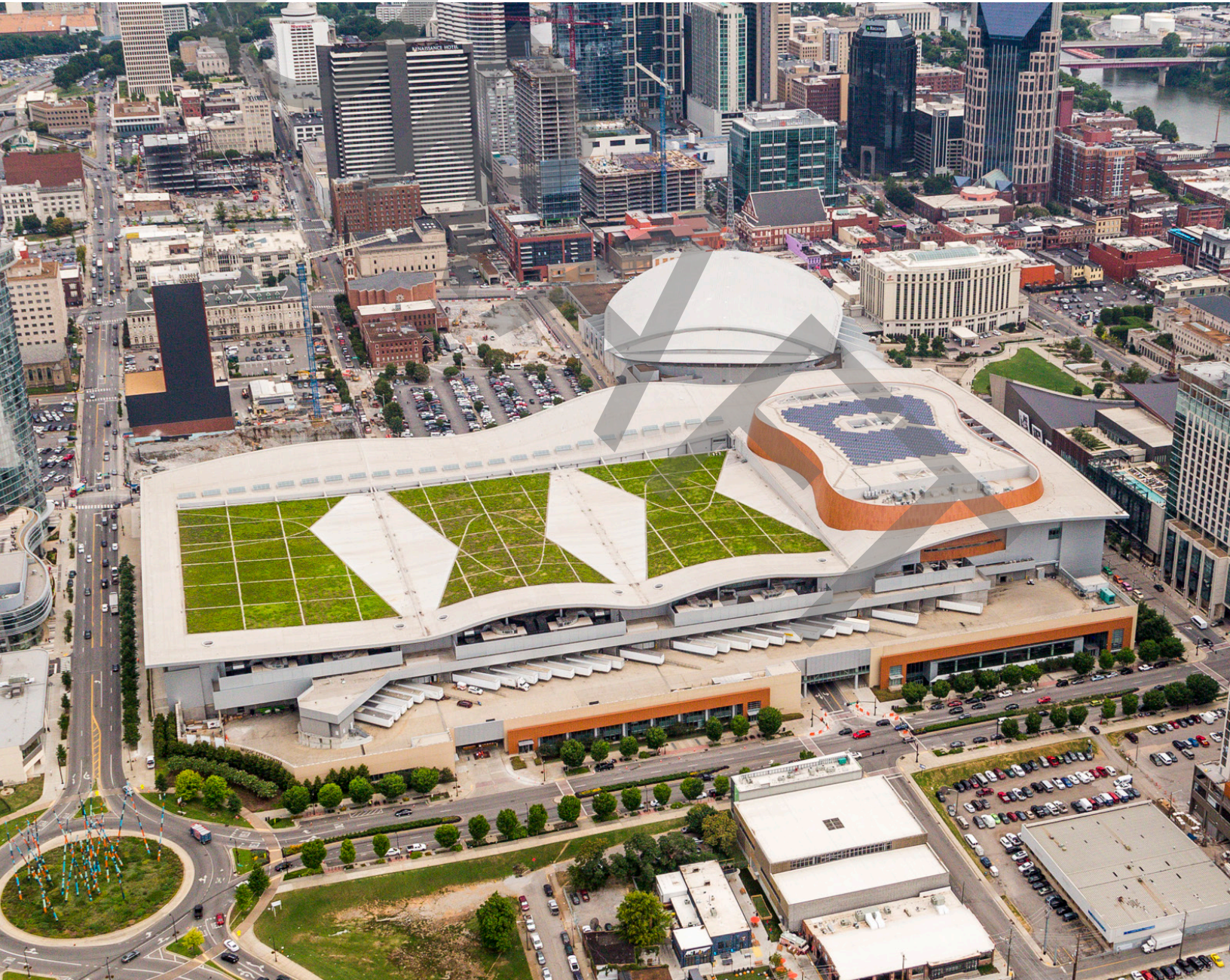
02D: Music City Center's (SoBro) four-acre green roof protects the expansive roof from harsh UV rays, wind, and stormwater runoff.
