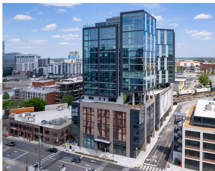
04A: Upper-level habitable liner buildings with residential uses, such as Prima at Paseo South Gulch (Gulch South), have program and activation along the perimeter of the above-grade structured parking garages.
