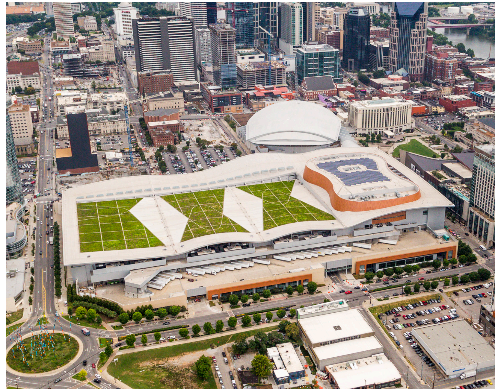
O2D: Music City Center's (SoBro) four-acre green roof protects the expansive roof from harsh UV rays, wind, and stormwater runoff.
