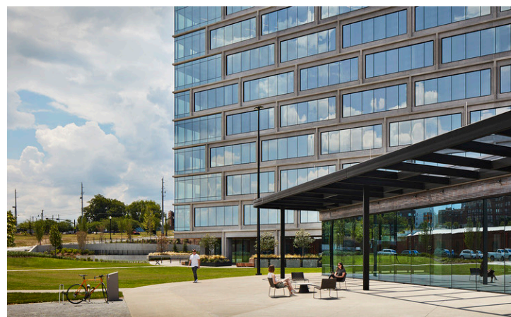
04B: Buildings with all parking underground – such as Peabody Plaza (Rolling Mill Hill) – create opportunities for integrated outdoor spaces.
