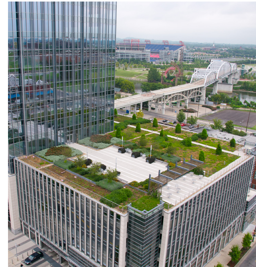
01C: Green roofs, like the one at The Pinnacle at Symphony Place (SoBro), can double as outdoor spaces for building occupants.
