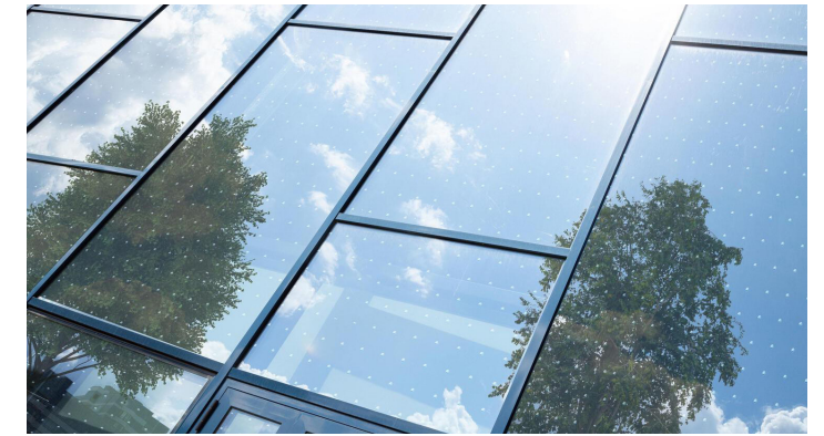
O2C: Glazing with contrasting patterns can help prevent bird mortality and increase energy efficiency in buildings.
