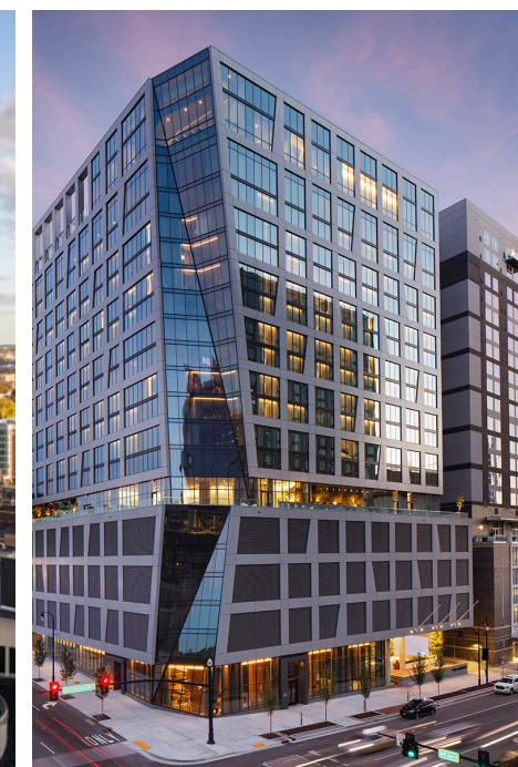
04E: A screening element features similar repetition and patterning to the glazing of the habitable levels at The Joseph (SoBro).
