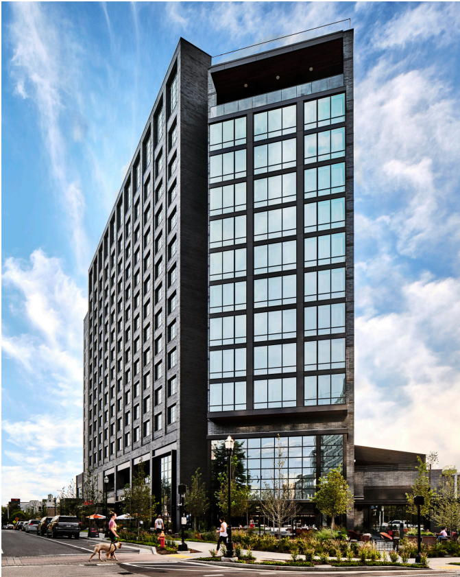
08C: The Virgin Hotel (Music Row) features a design that responds to its context at a major intersection. It presents a unified aesthetic between its lower levels and their relationship to the human scale and the upper floors, through clear massing, articulation, and fenestration.
