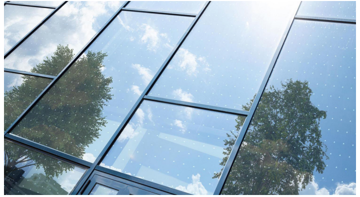
02C: Glazing with contrasting patterns can help prevent bird mortality and increase energy efficiency in buildings.
