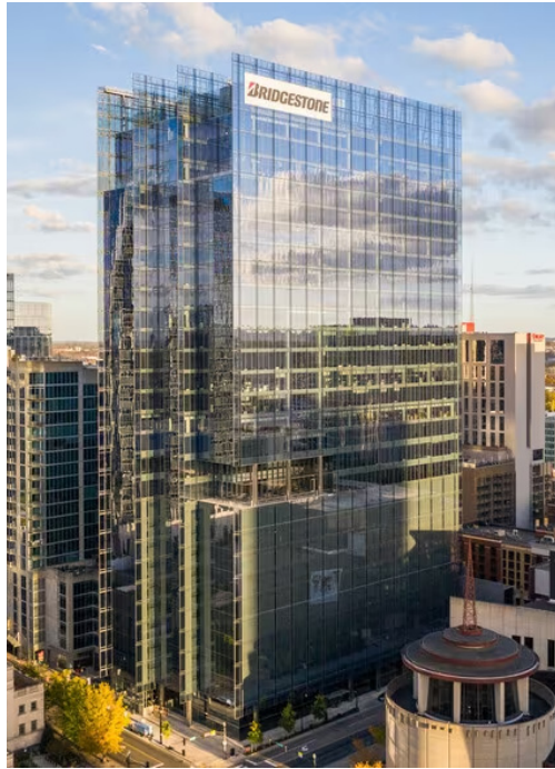
04D: Parking levels, at the Bridgestone Tower (SoBro) are screened from view with materials that fit seamlessly into the tower design.
