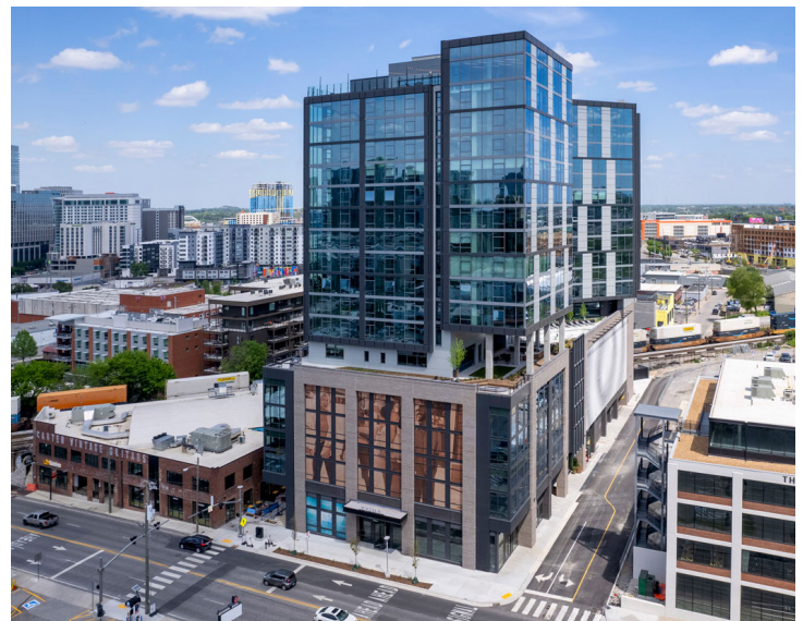
04A: Upper-level habitable liner buildings with residential uses, such as Prima at Paseo South Gulch (Gulch South), have program and activation along the perimeter of the above-grade structured parking garages.
