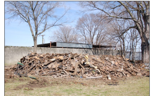
Below: After demolition.
