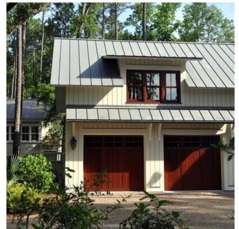
Examples of appropriately scaled outbuildings.
