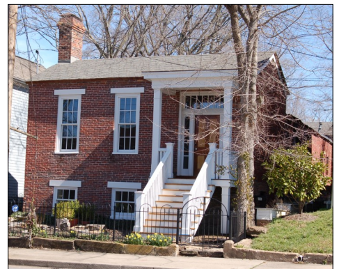
One of Germantown’s oldest residences (c. 1840) on Fifth Avenue North during a renovation.
