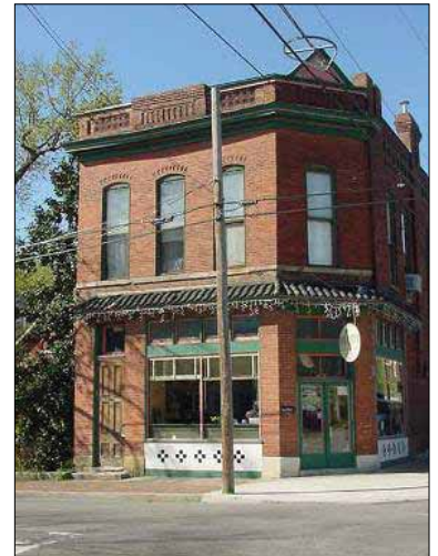
The Neuhoff store has been renovated and operated as a restaurant since the 1980s.
