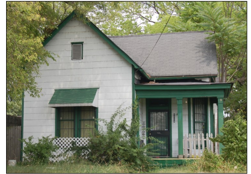
Above: Prior to demolition.
