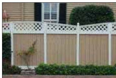
Examples of privacy fencing on side or rear lot lines.
