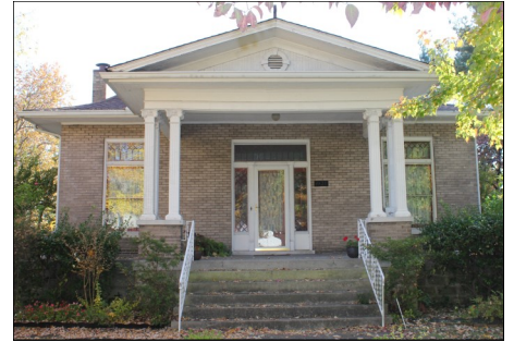
1128 Greenfield exemplifies modest Neoclassical applications represented in Inglewood Place.
