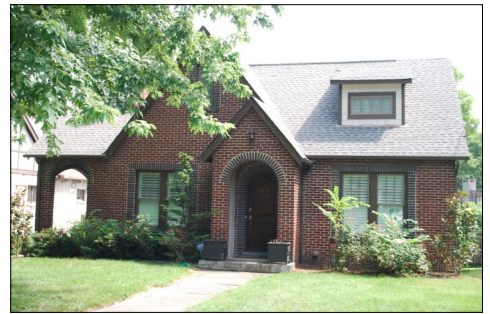
179 Kenner Avenue was designed in the Tudor Revival style.
