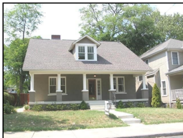
Side gable with full width porch at 1617 5th Avenue North.
