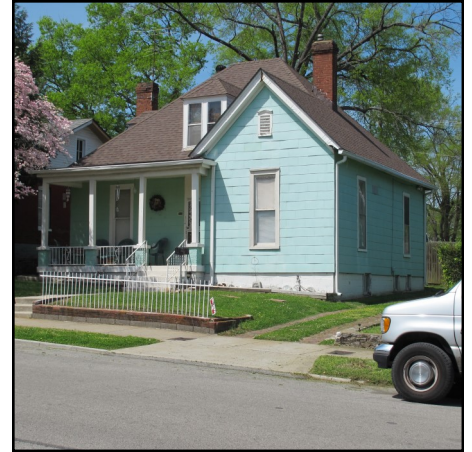
912 Gilmore is a Victorian-era building.
