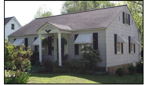
3518 Kennedy is an example of the Colonial Revival style applied to a Minimal Traditional residence.
