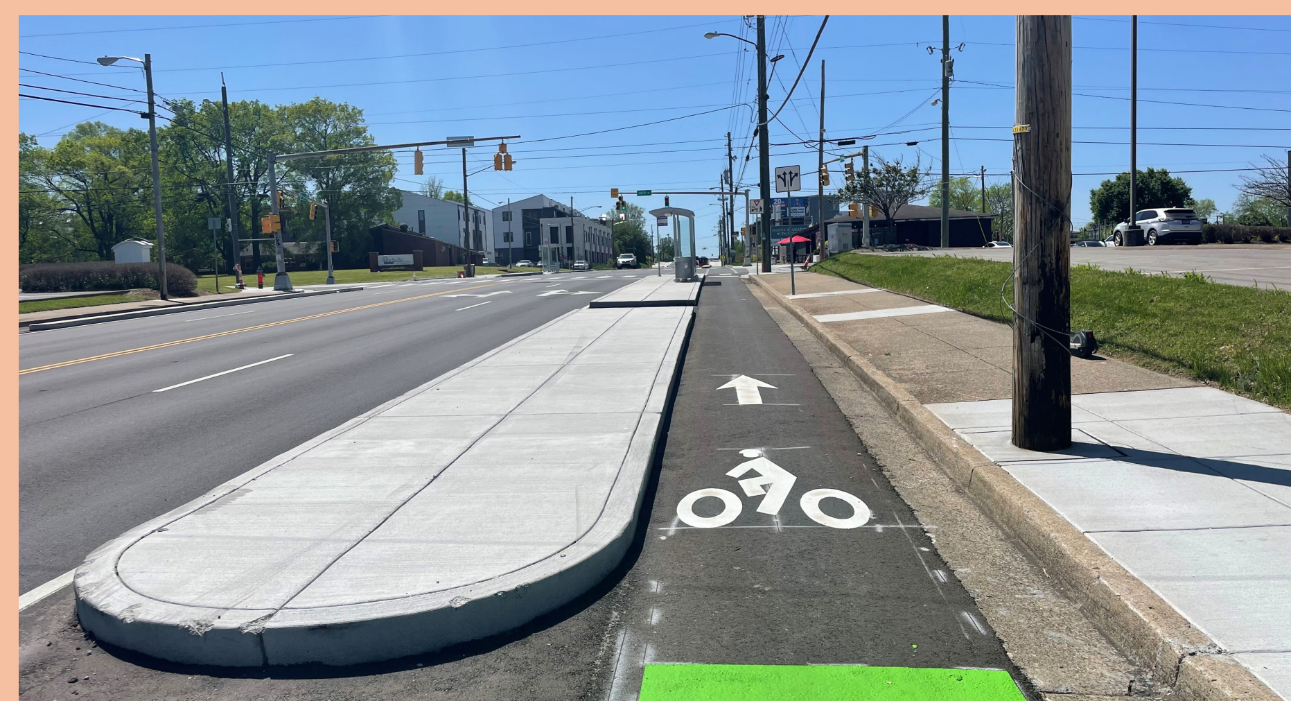
Typical buffered one-way cycle track 12 th Ave South, Nashville
