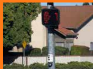
Accessible pedestrian-activated flashing lights and countdown timers
