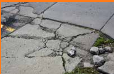
Repairing cracks or broken ramps
