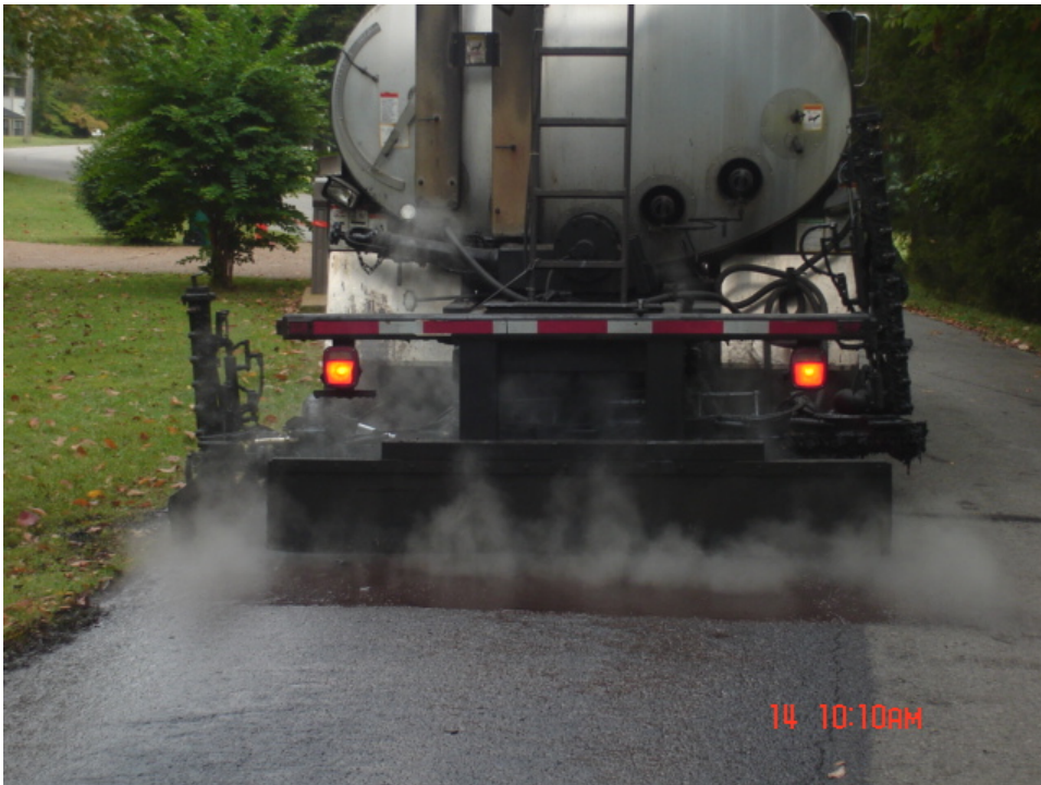
Figure 8.2. Application of PASS surface sealer on Metro street.
