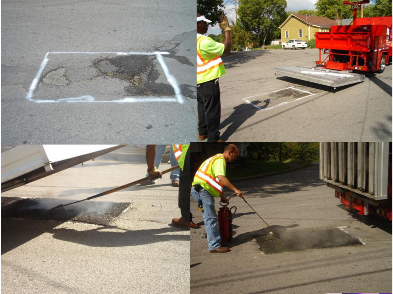
Figure C.24. Heating area to be patched with Infrared machine.
