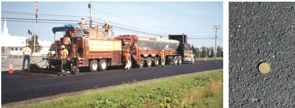
Figure C.7. Truck-mounted self-propelled micro-surfacing machine (left) and finished surface using Type II aggregate (right).
