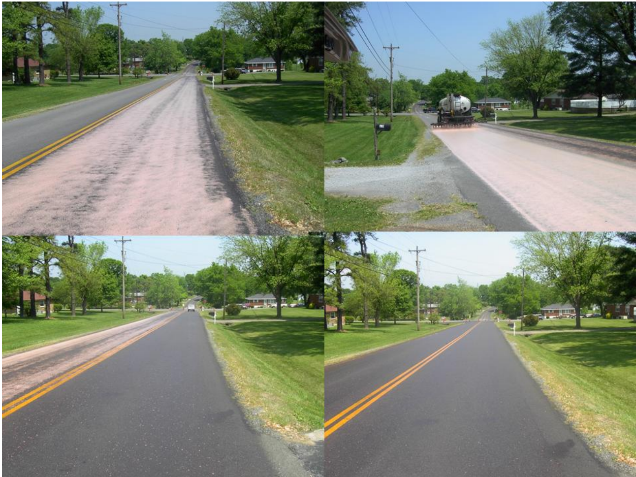
Figure C.20. Reclamite application on field section in Nashville.
