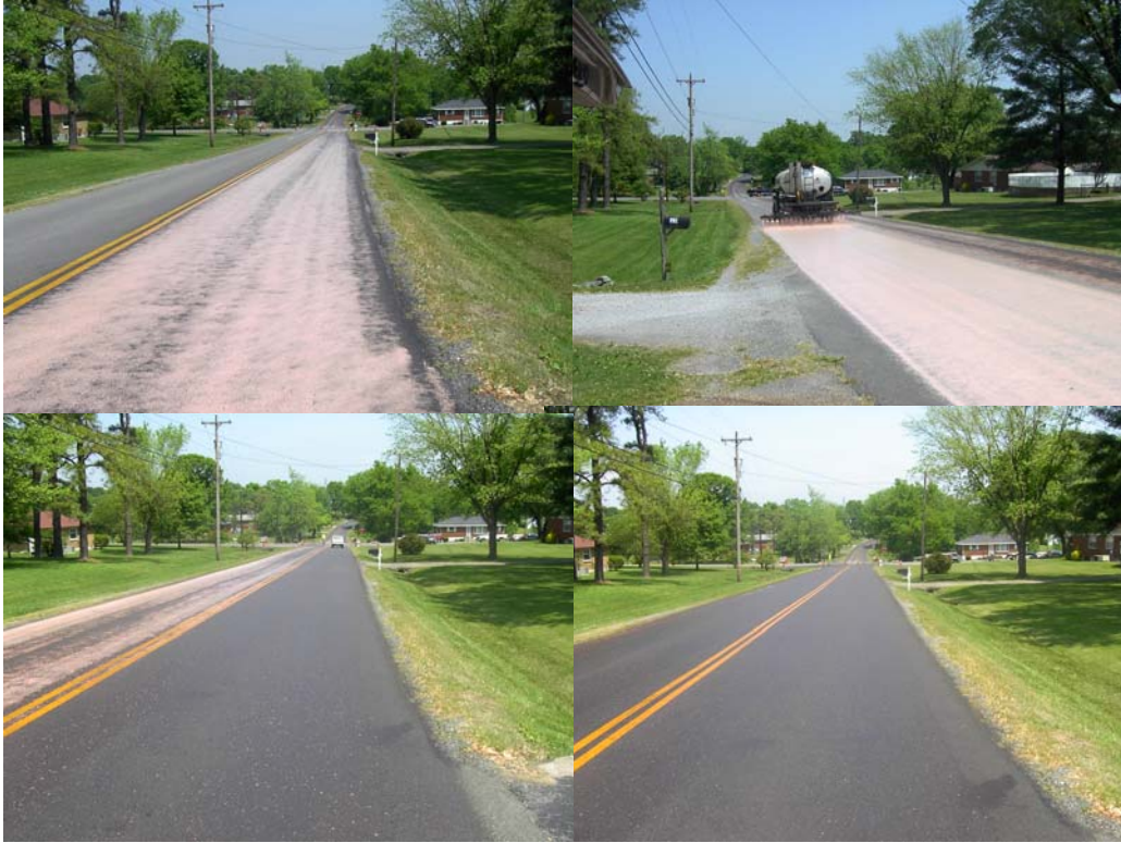
Figure 8.1. Application of Reclamite to Metro street.
