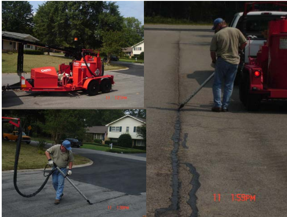
Figure 8.3. Crack sealing of Metro streets.
