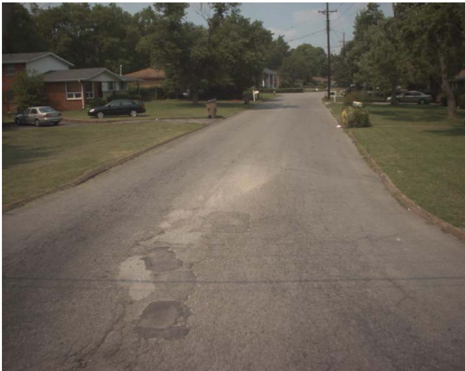
Photo 4.3. Tanglewood Trail, segment 8108, fatigue cracking, roughness, and patching.
