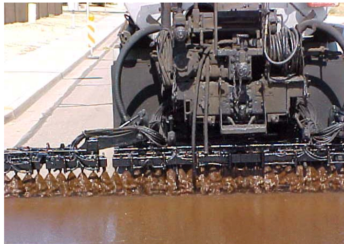
Figure C.11. Asphalt distributor applying emulsion.
