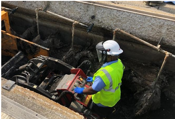
Images from the Dry Creek Water Reclamation Facility Channel Cleaning (Summer 2023) depicting the accumulation of flushable wipes along aeration lines in Primary Treatment.
