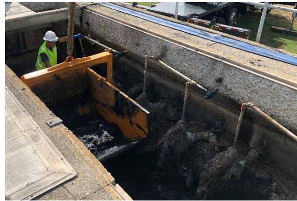
Images from the Dry Creek Water Reclamation Facility Channel Cleaning (Summer 2023) depicting the accumulation of flushable wipes along aeration lines in Primary Treatment.
