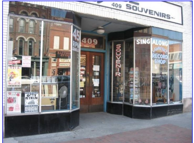
Historic storefronts such as this ca. 1930 design with Carrara glass at 409 Broadway should be retained and, if needed, repaired using materials that match the historic materials.
