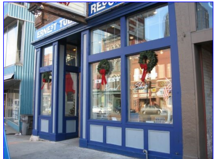
This modern storefront appropriately replicates the missing historic storefront through its incorporation of the typical storefront elements of a recessed entryway, wood-paneled bulkheads, clear glass display windows with wood frames, and clear glass transoms with wood frames. 615-862-7970
