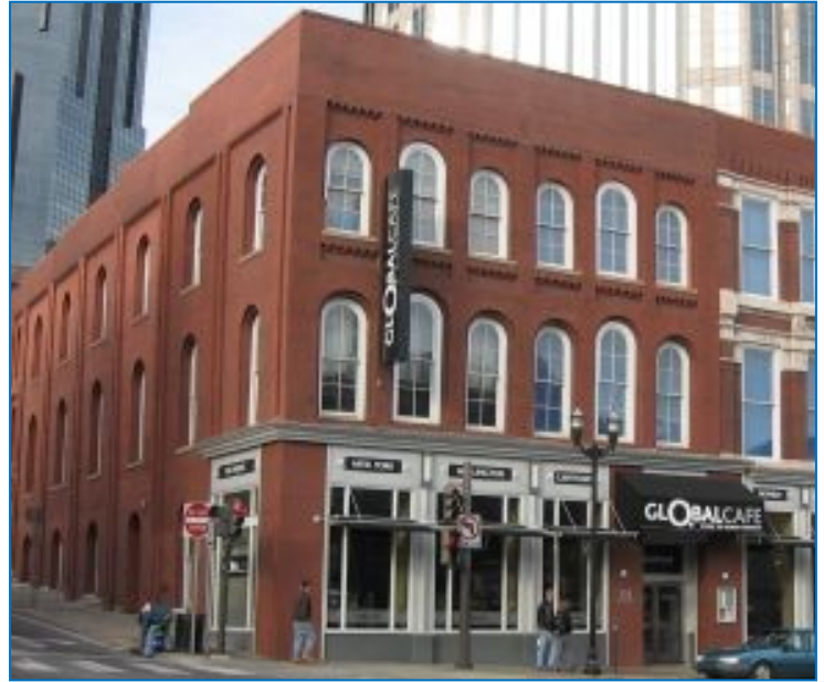
Historic masonry should not be concealed or obscured.
