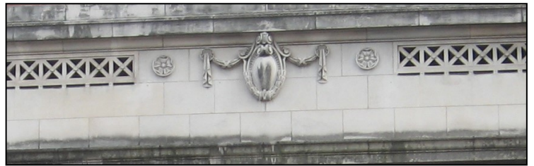
Historic cast concrete highlights the American Bank Building at 301 Broadway.
