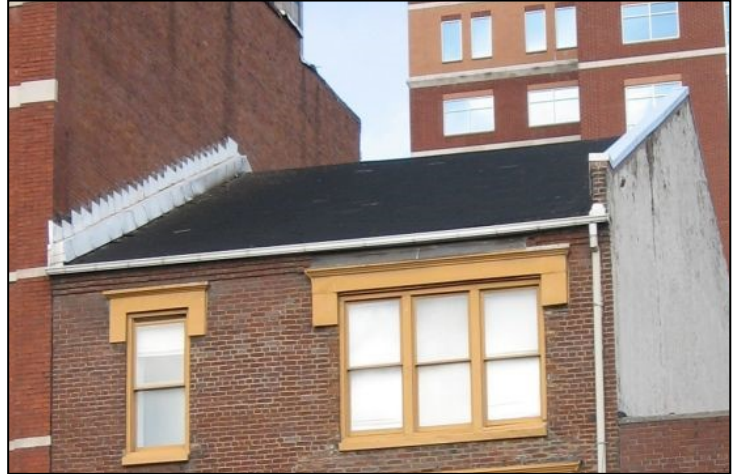
The gabled pitch of this roof is unusual in the district. Its historic pitch and appearance should be retained.
