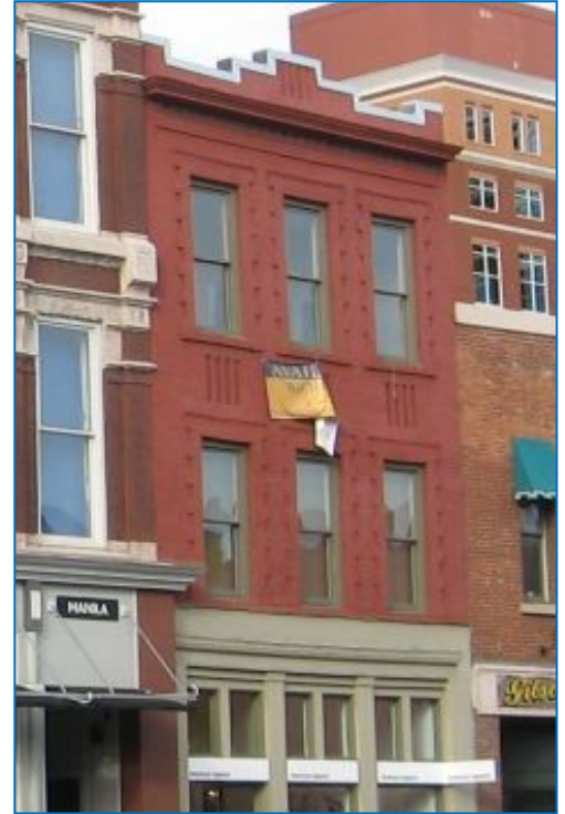
Masonry painted for preservation purposes should use a brick-colored paint.
