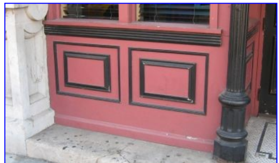
The painted, paneled wood is an appropriate modern bulkhead design. 615-262-7970
