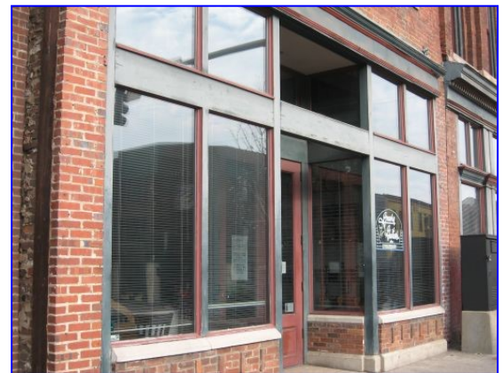
Modern display windows at this storefront are appropriate in their size, placement, clear glass and painted wood materials.
