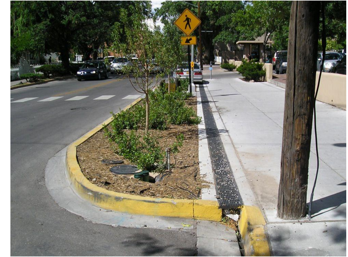
Concrete Curb Extension Example
