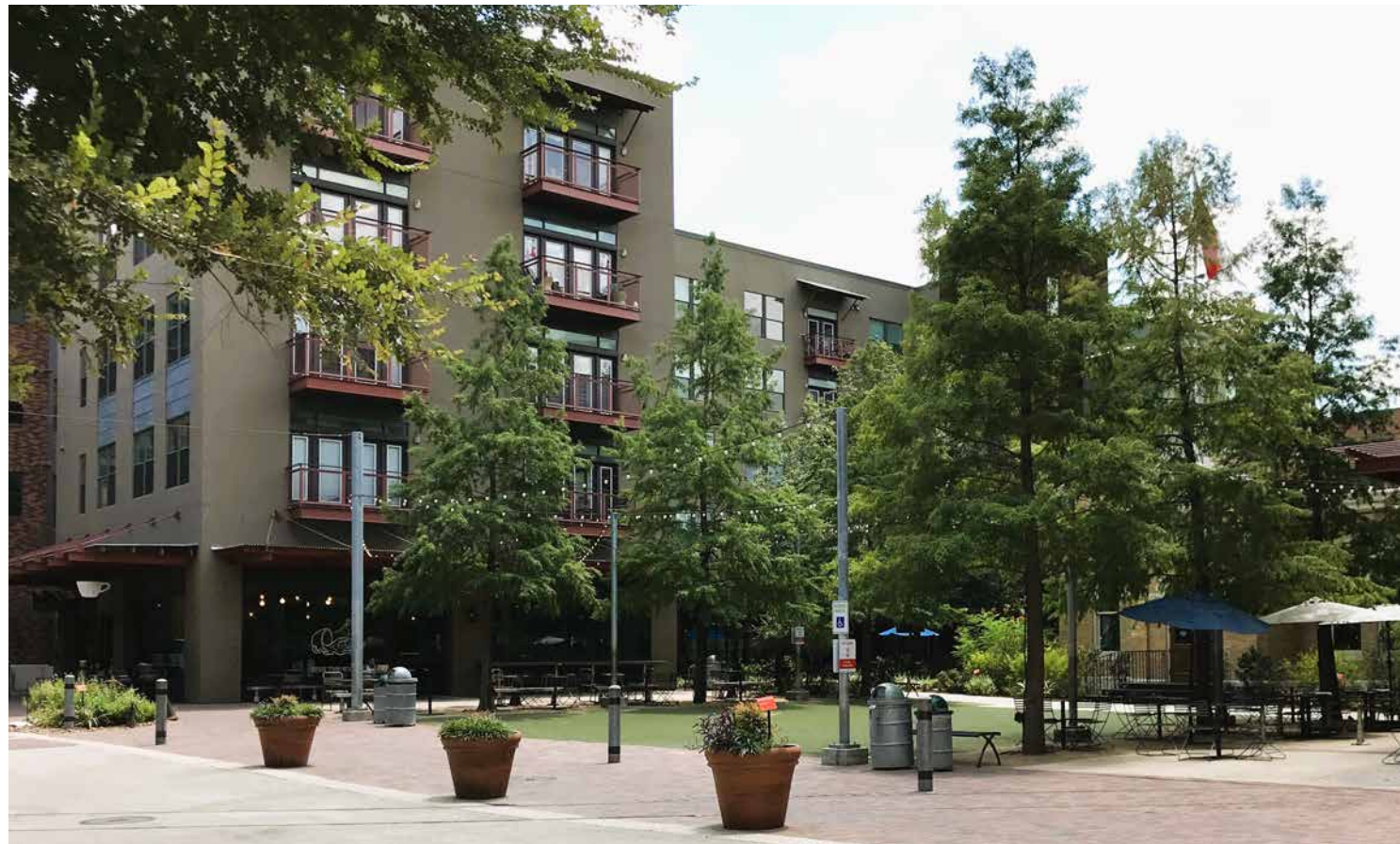
A mixed-use, mid-rise building illustrates articulated massing and change in building materials.
