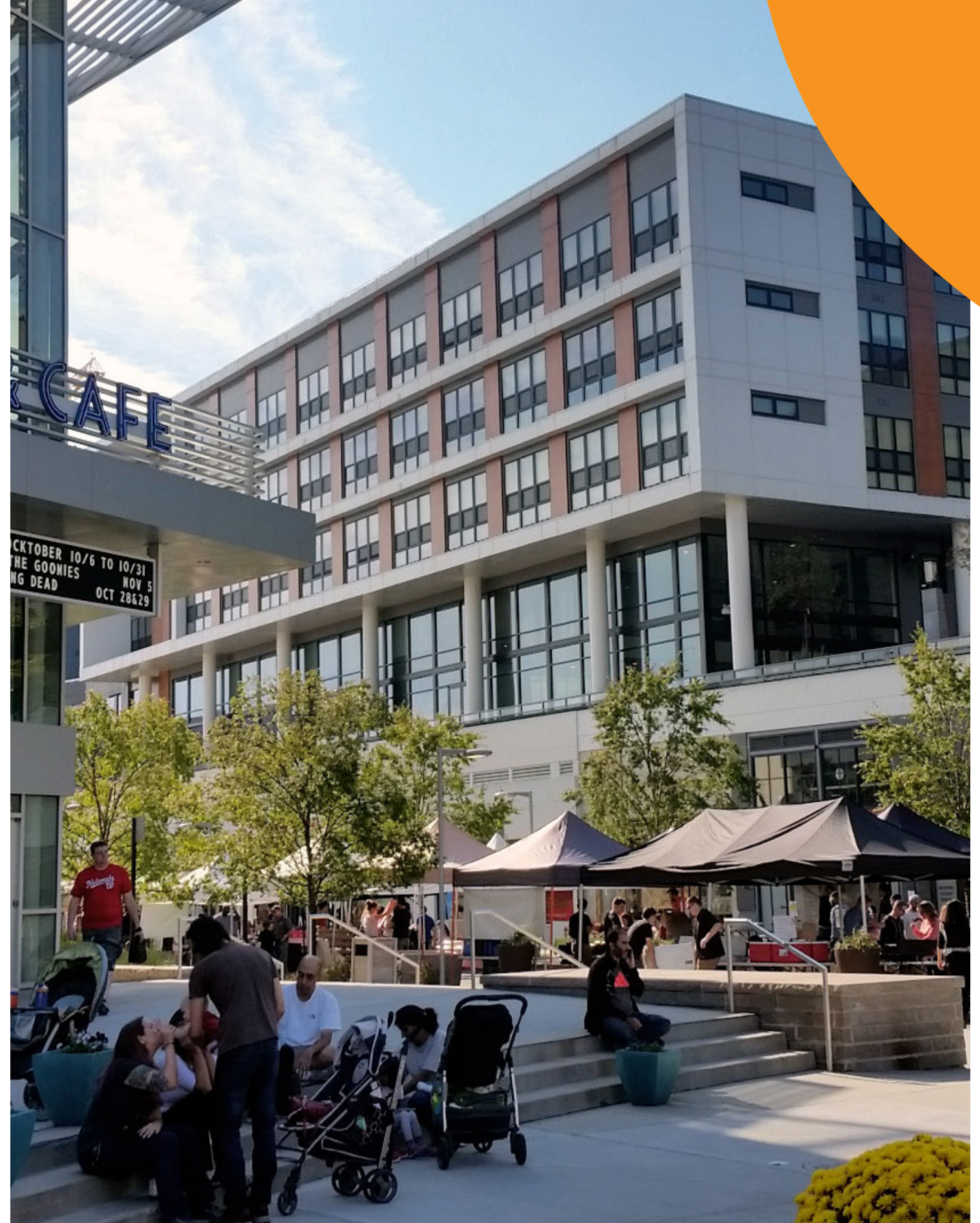
Fig. 1-11. Future development on the Global Mall site should emphasize an inviting and safe public realm with a range of open spaces for people to gather.
