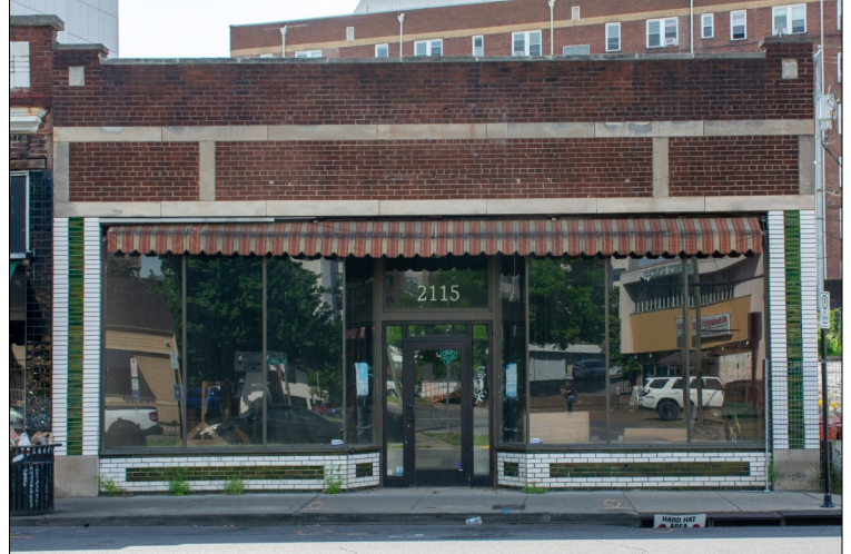
Glazed brick of white and green and stone details are character defining features of 2115 Elliston Place.
