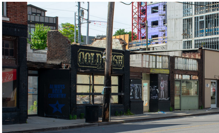
Doors and windows were replaced prior to designation but the dimension and design of entries should be retained.
